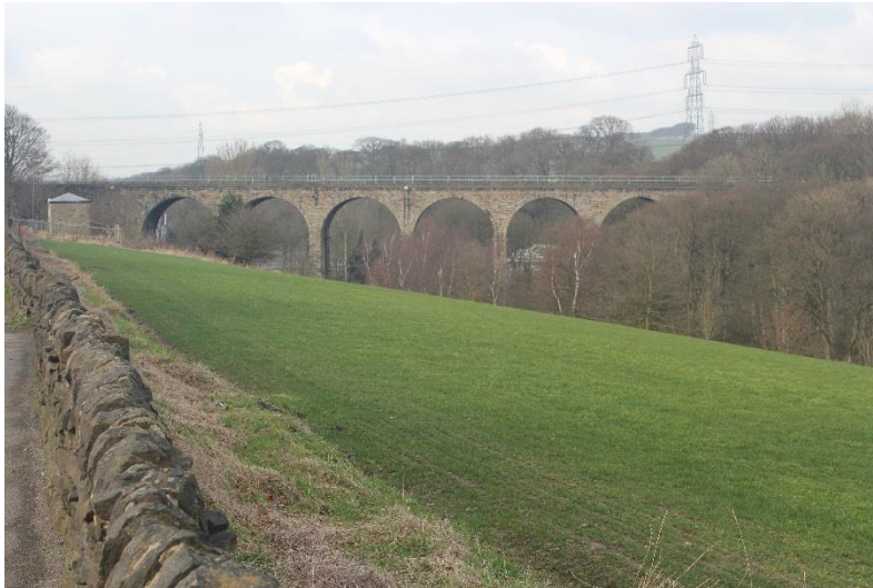
View of Viaduct, Sheffield Road opposite Eddyfield
