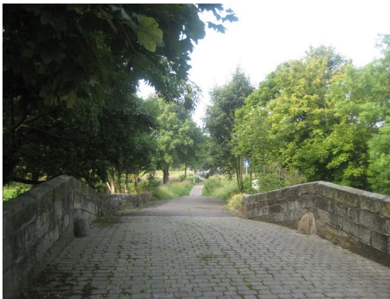
The Old Oxspring Road Bridge
