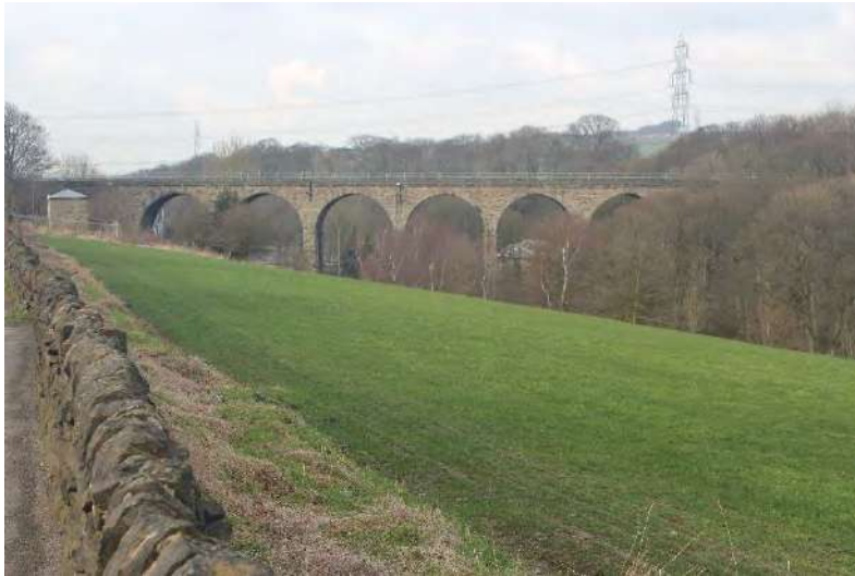
View of Viaduct, Sheffield Road opposite Eddyfield
